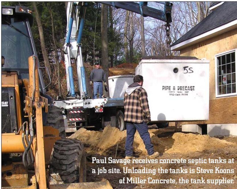
Paul Savage receives concrete septic tanks at a job site. Unloading the tanks is Steve Koons of Miller Concrete, the tank supplier.
