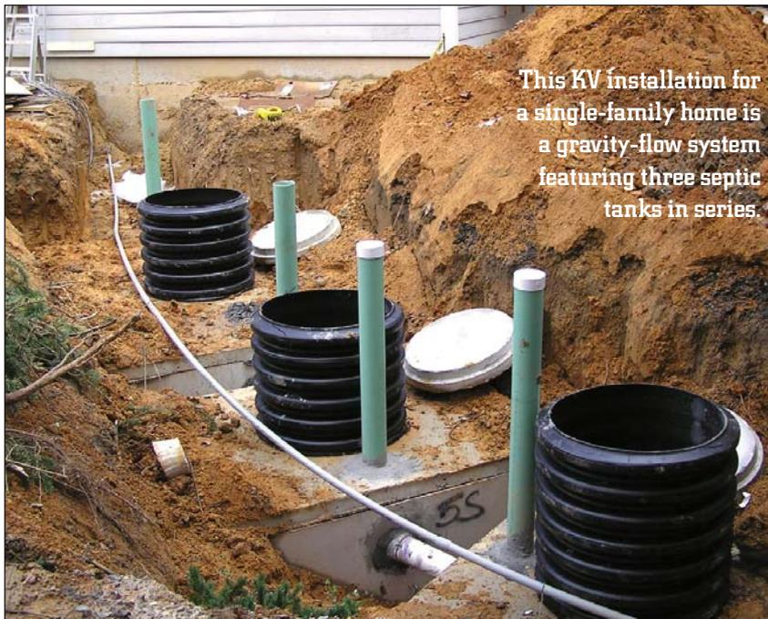
This KV installation for a single-family home is a gravity-flow system featuring three septic tanks in series.
